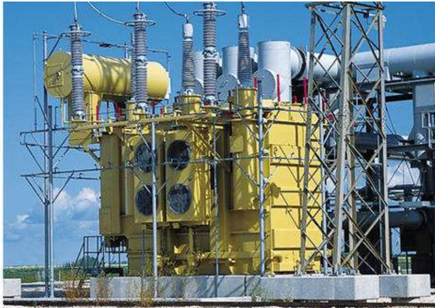
Fig 2.4 Converter transformer
